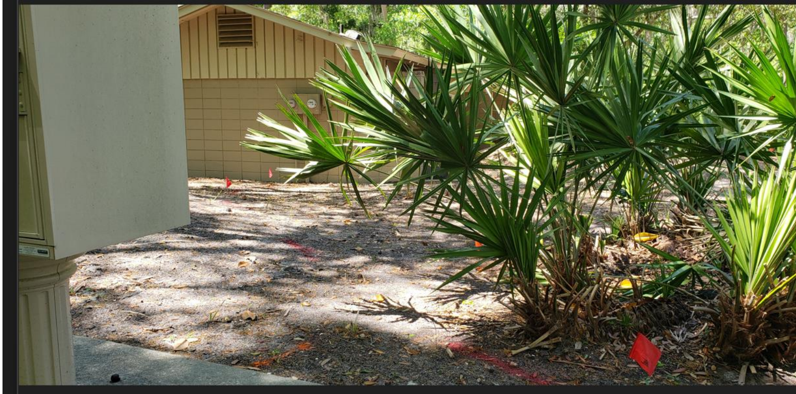
Electric to G Building
